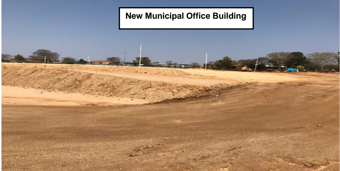
Construction of New Municipal Office Building
