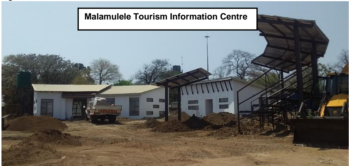
Construction of Malamulele Tourism Information Centre
