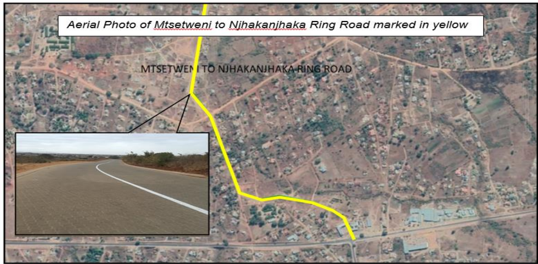
Upgrading of Mtsetweni to Njhakanjhaka Ring Road Phase 2
