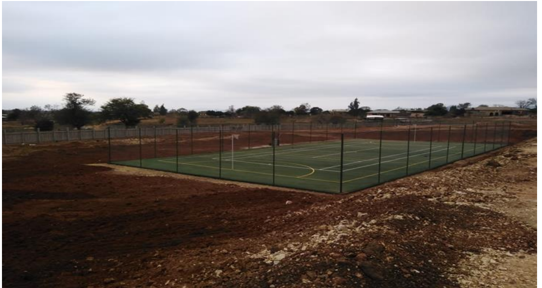
Picture 13 Construction of Davhana Stadium Phase 1
