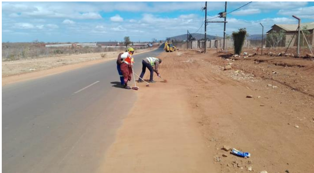
Upgrading and Construction of 7,7km Rural Road from Gravel to Tar
