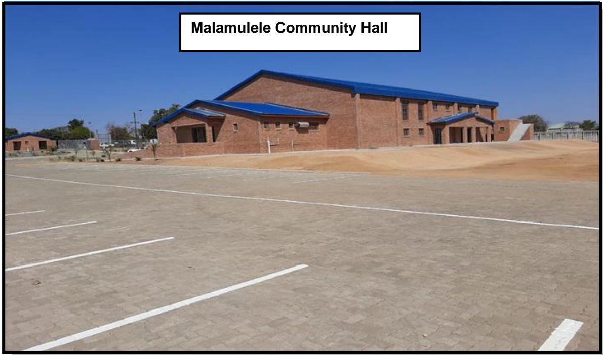
Construction of Malamulele Community Hall
